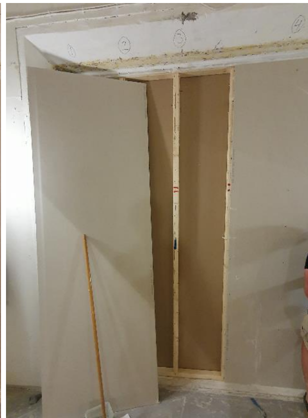
Figure A4.8: M3 and M4 during construction.
