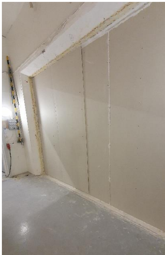
Figure A4.9: M4 during construction.
