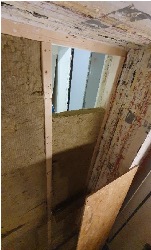
Figure A4.3: Test wall M1 during construction.
