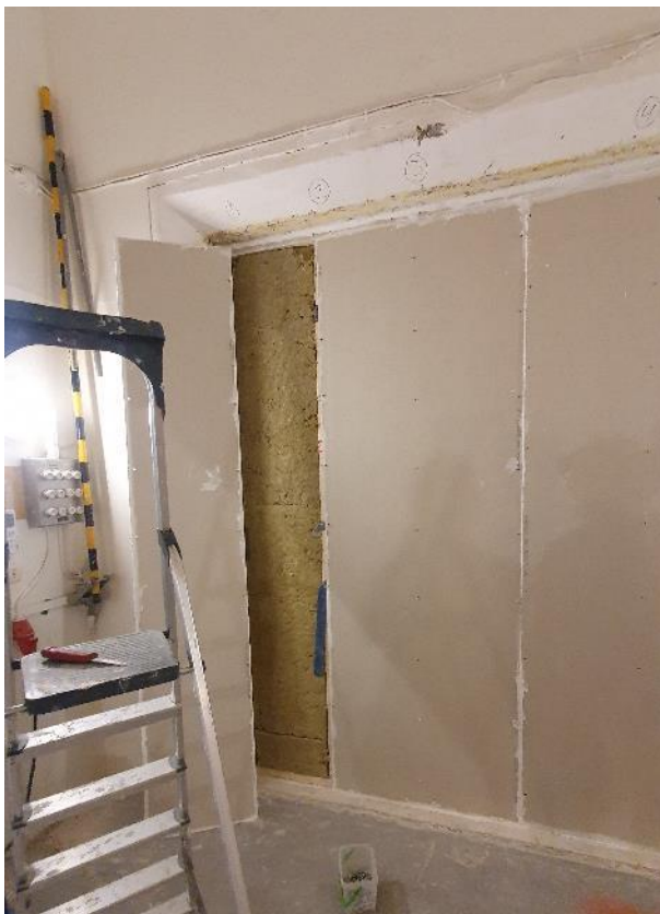
Figure A4.7: M2 during construction.
