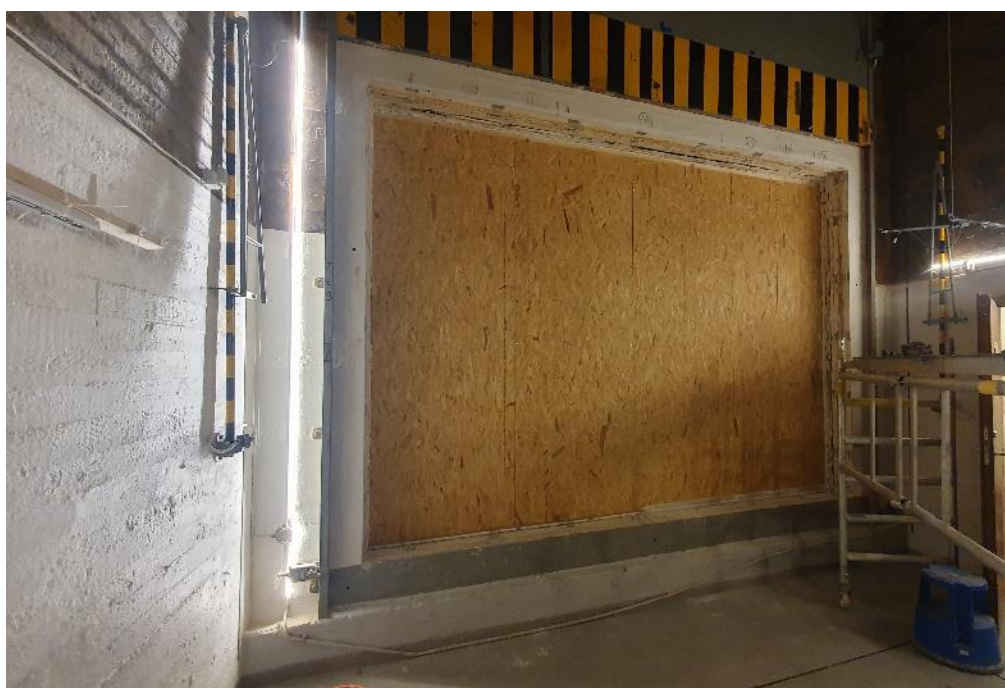
Figure A4.2 Test wall M1 during construction.
