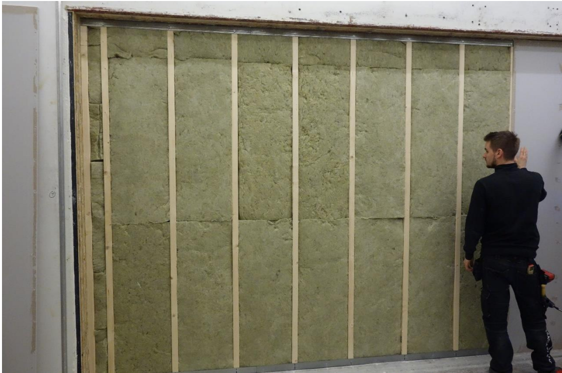
Picture 1 – The wall during mounting.
