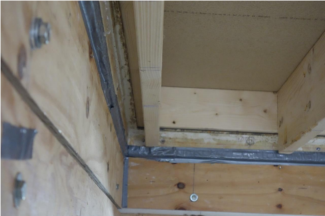
Picture 8 – The wooden studs on the short side, 45x145 screwed into 45x220.
