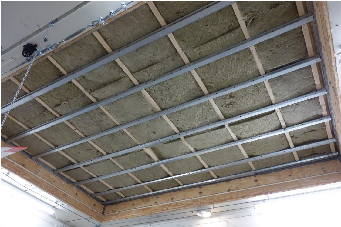
Picture 4 – The floor from below with the Knauf AP Acoustical stud.
