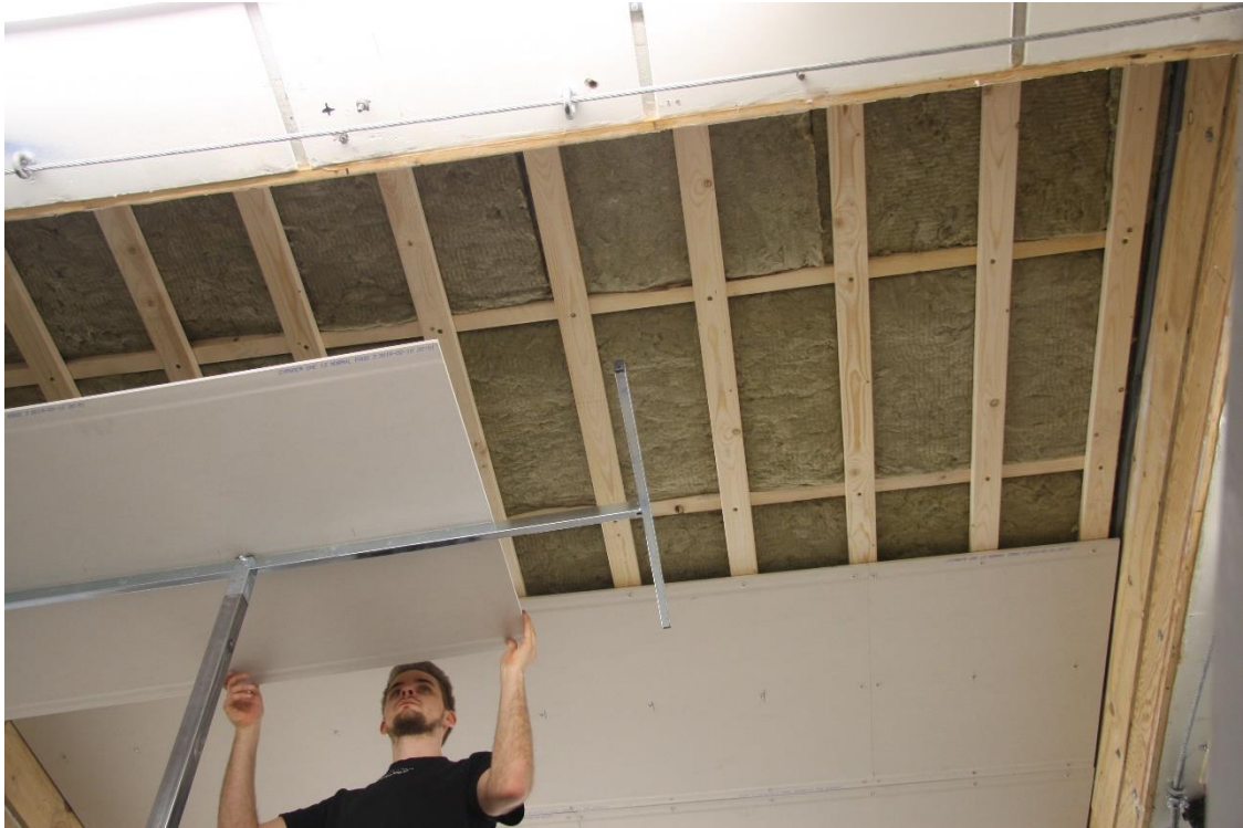
Picture 2 – The floor from below. The furring 28x70 can be seen.
