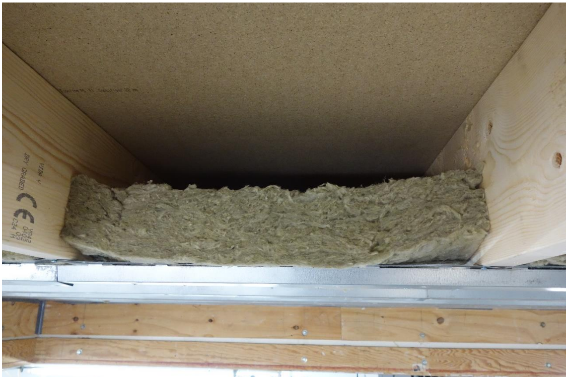
Picture 5 – The mineral wool between the wooden studs 45x220.
