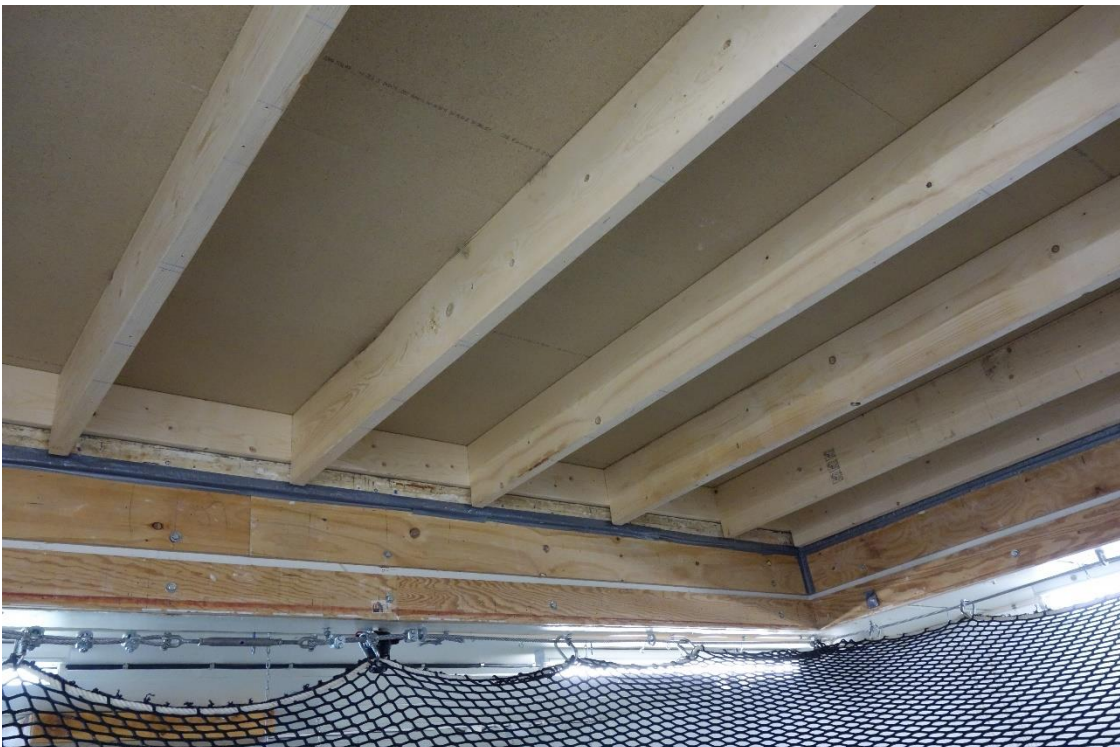
Picture 7 - The wooden studs 45x220 where attached by screws into studs 45x145 placed directly on the edges of the test opening on all sides.
