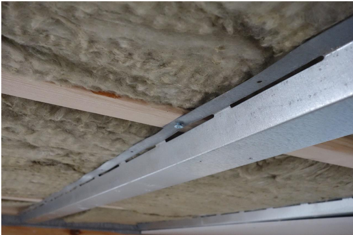
Picture 3 - The Knauf AP Acoustical stud.
